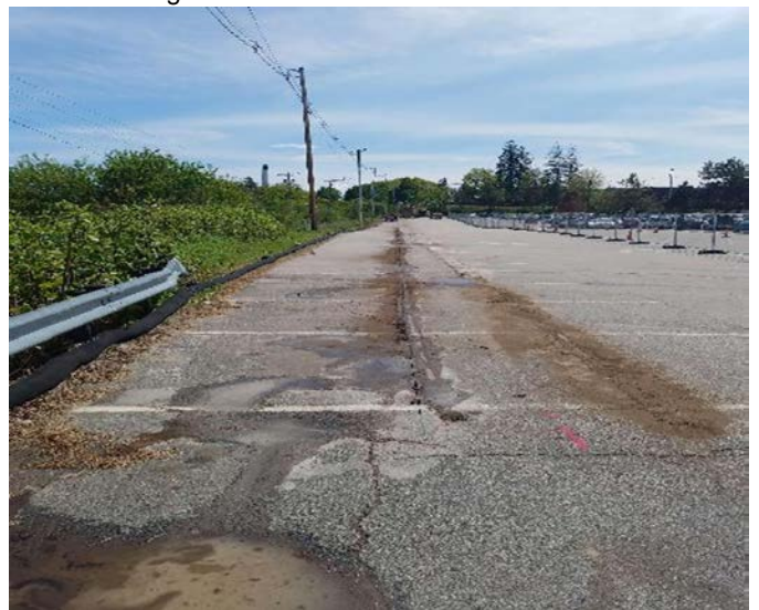
Fig 8: McCourt saw cutting A lot. Viewing south.
