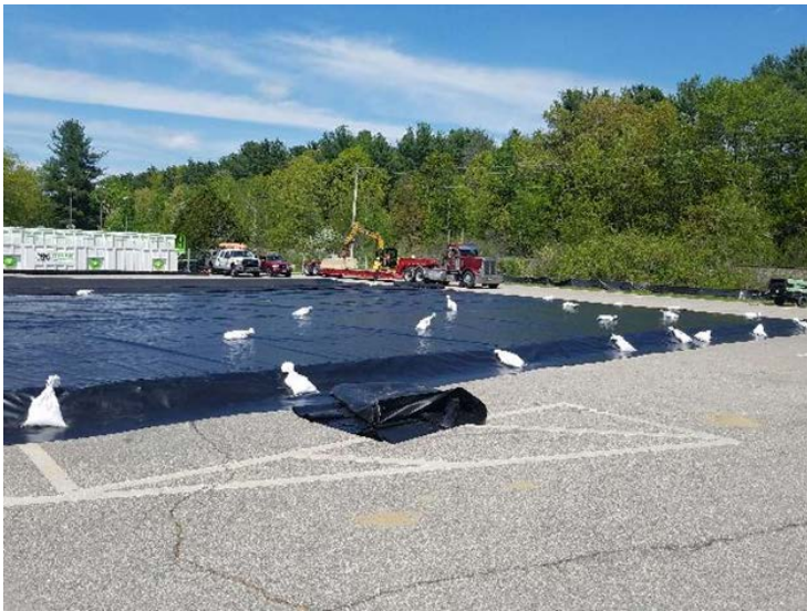
Fig 7: Strategic setting up soil stockpile area in A lot. Viewing northeast.
