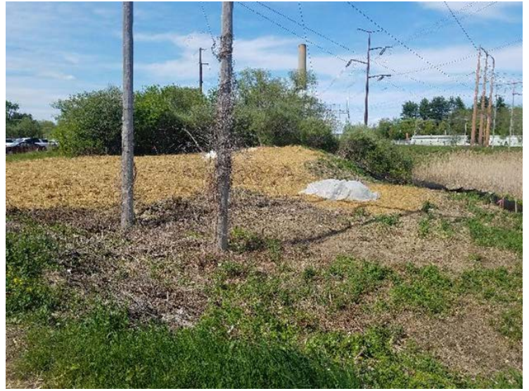
Fig 6: JRC finished removing timber matting & scattering straw over exposed soil around Str. E194-7 & F107-137. Viewing north.
