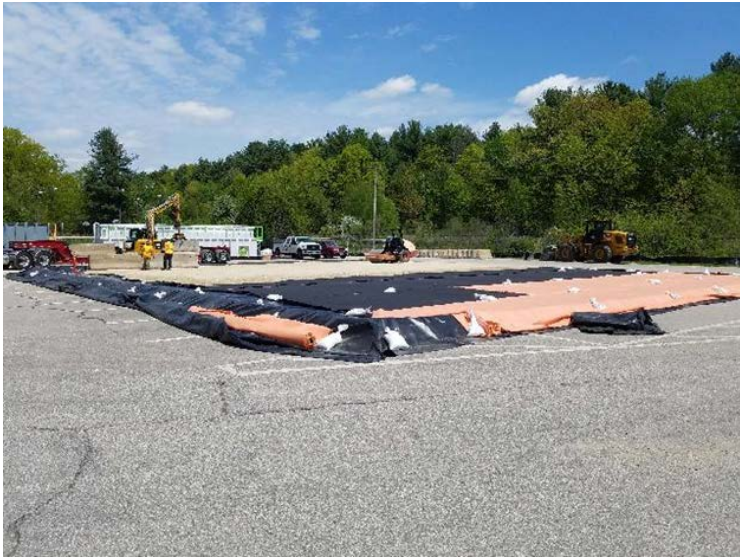
Fig9: Soil stockpile area in A lot. Viewing northeast.
